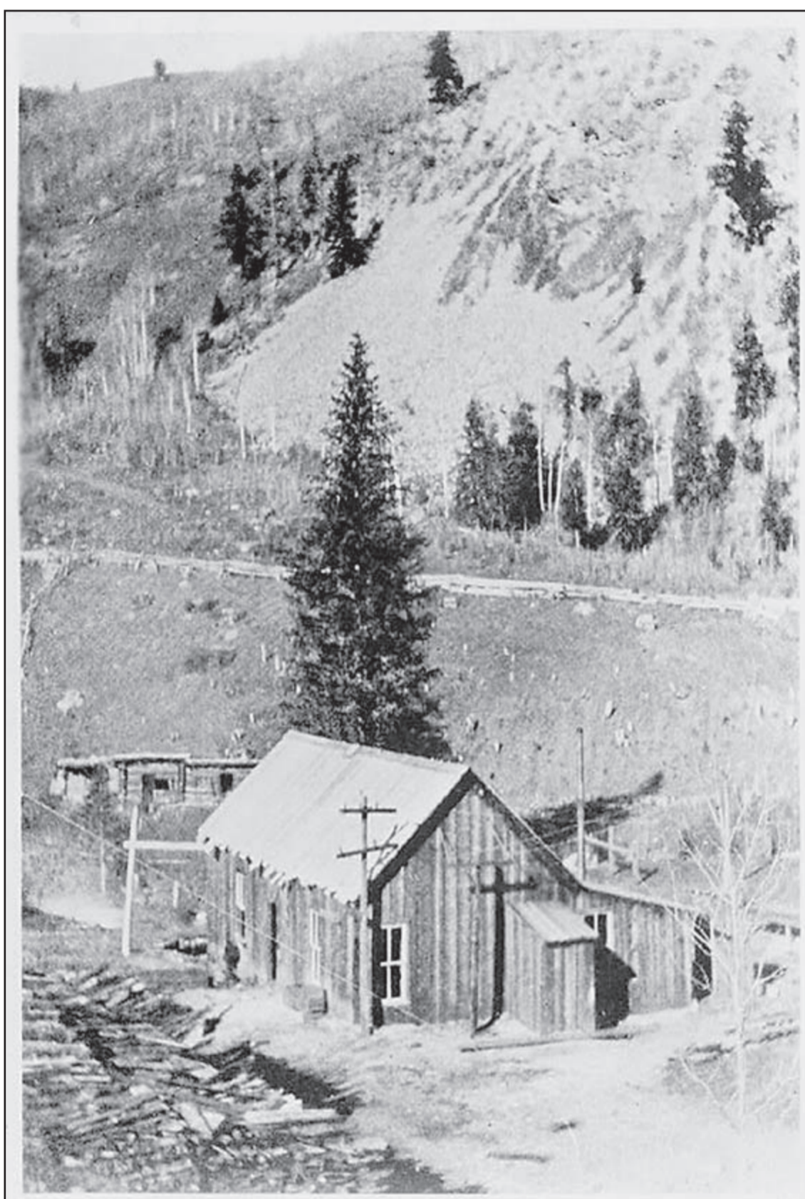
The Ames Power plant near Ophir as it appeared about 1894, three years after it was put into operation. (Library of Congress)
