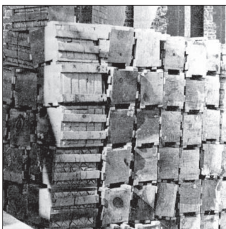
Crates of bricks are stacked in Vernal, Utah, during construction of the Coltharp Building.
