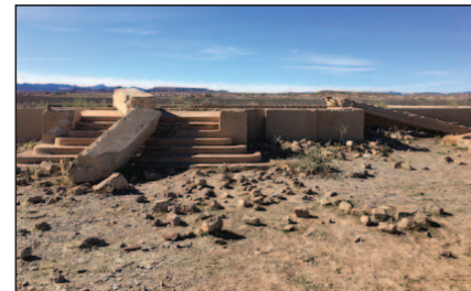
The foundation, steps and fallen pillars are all that remains of the St. Thomas School in 2020.
